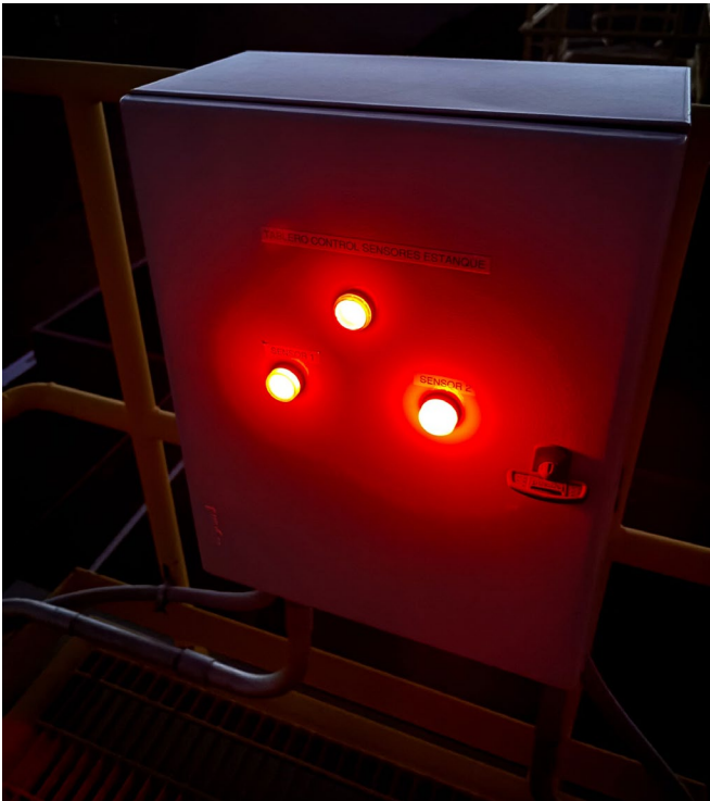
Fig. 16. Top: Panel pilot lights at the Simons Observatory. Bottom: Effects of red pilot lights on a panel near an antenna at the future GMT site. Their luminous impact is visible in medium-exposure images. This sector is adjacent to where the OPCC conducts sky quality measurements.
