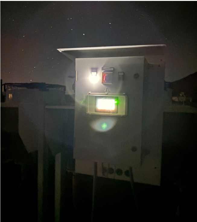
Fig. 16. Top: Panel pilot lights at the Simons Observatory. Bottom: Effects of red pilot lights on a panel near an antenna at the future GMT site. Their luminous impact is visible in medium-exposure images. This sector is adjacent to where the OPCC conducts sky quality measurements.
